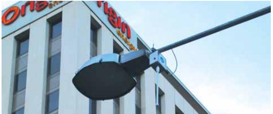
Installations like these require people with cabling and electrical skills. The nodes on the poles are powered by the electrical service on the light pole itself.
