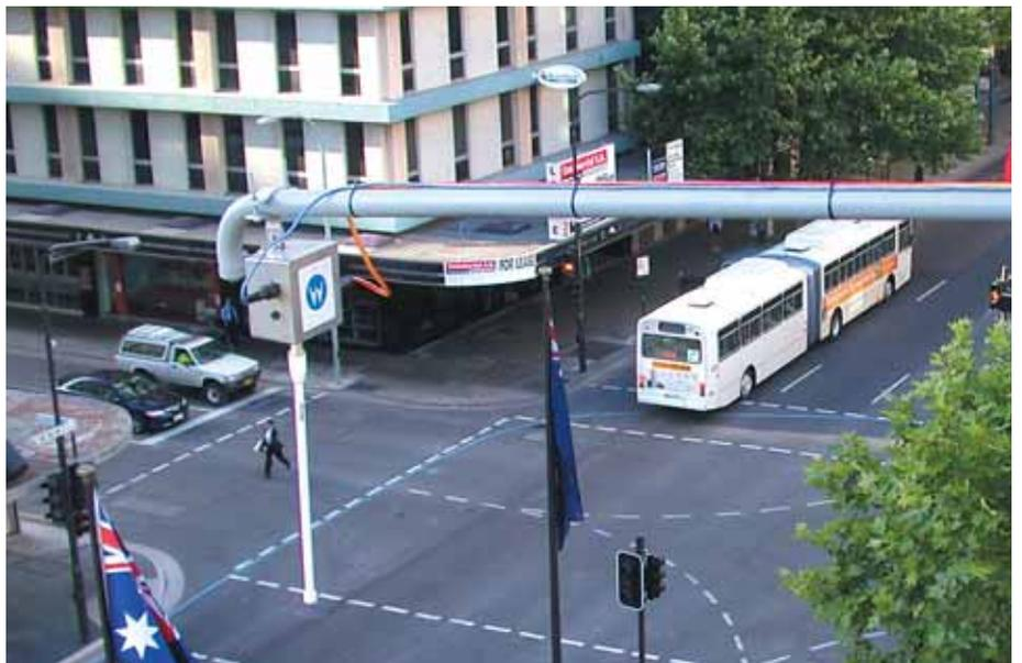
Mesh networking uses wireless nodes, like this one hanging from a pole, to provide wireless LAN coverage and wireless backhaul. The nodes interconnect to form a self-healing network or mesh that can support mobile data access, voice, cameras down a street, around a campus or over a whole city or community.
